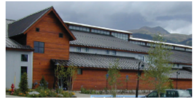
Height variation may occur with changes in wall heights for different building modules.
