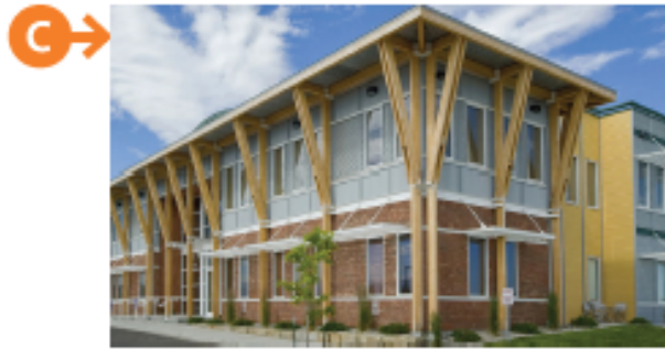
Integrate architectural details with facade articulation. Use exposed posts, beams, trusses and brackets, for example.
